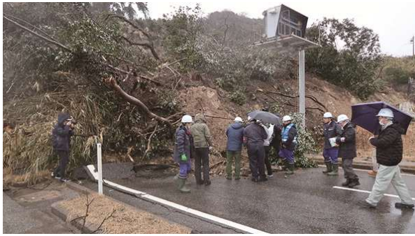
Photo 2 Maura-machi, Suzu-shi (location of large-scale collapse near Osaka Tunnel, National Highway No. 249)
