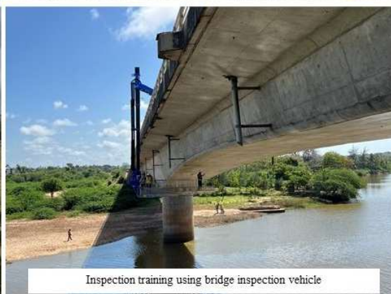
Setting up traffic restrictions and bridge inspection vehicle
