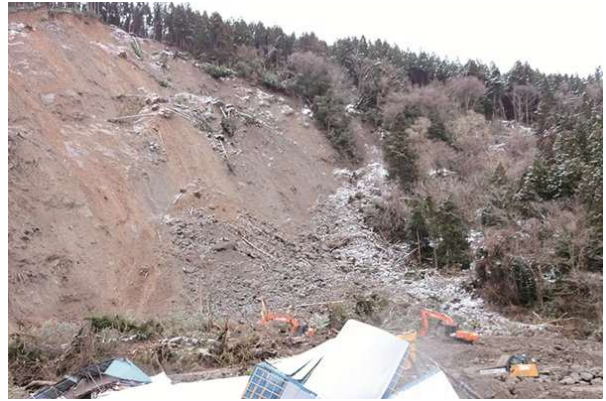
Photo 3 Kumano-machi, Wajima-shi (location of Kawaradagawa River channel blockage and landslides across a wide area, including locations that had been restored from the earthquake that struck in 2007)
